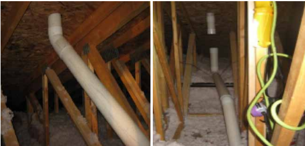
Figure 11. Example of Radon Pipe Positioned on Angle Figure 12. Example of Radon Pipe Cut and Straightened
