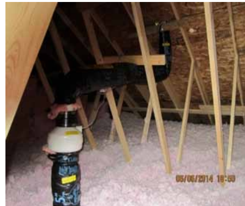
Figure 4. Example of Insulated Pipe
